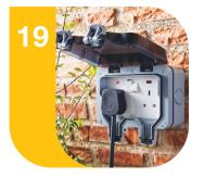
If you use gardening tools, make sure that the outdoor sockets are suitable for outdoor use and that they are protected by a Residual Current Device (RCD 30mA).
